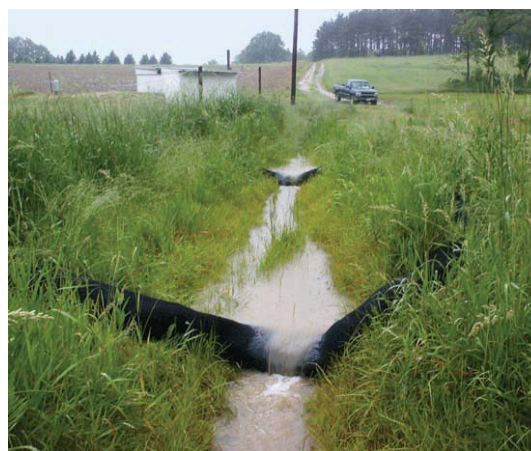
Runoff from a field planted with corn is directed into a grassed waterway where it passes through and over a series of compost-filled filter socks that help reduce levels of nutrients and herbicides.
