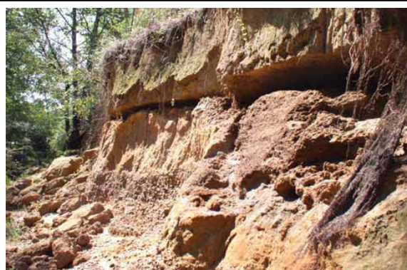
An example of seepage erosion from a section of Goodwin Creek, Mississippi.
